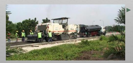
Single-Unit Train -Pulverizes, adds Recycling Agent Based on RAP Weight, Mixes Materials, Places CR Mixture.
