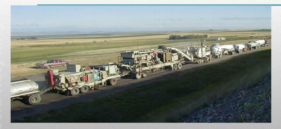
Multi-Unit Train Pulverize, Screen, Crush, Add Recycling Agent Based on RAP Weight & Mix in Pugmill
